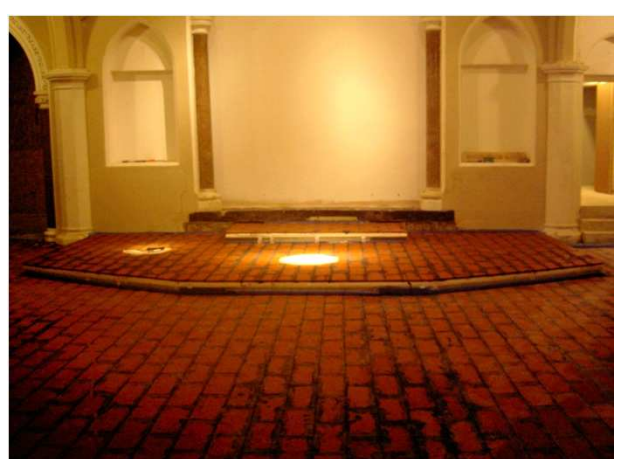
Screed Replacement Tiles installed in preparation for carpet and natural slate finish.
