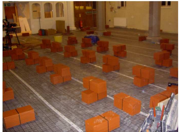
Screed Replacement Tiles are laid out in piles prior to installation.
