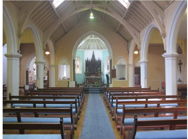
Interior of the church before reordering. Existing floor constructed from concrete slab. Slab was too poor to save so new one was cast.
