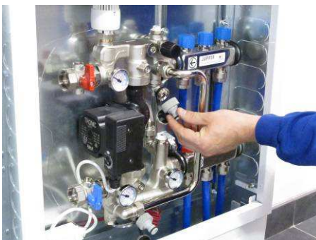
Attach hose lock adapters to upper and lower valves
