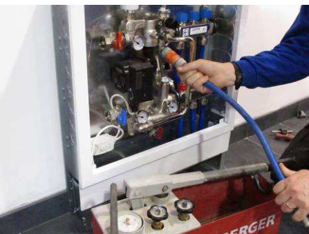
Re-open all blue caps on upper manifold prior to pressure testing. Connect pressure test equipment to upper return valve. Before connecting pressure test to the in-situ hose lock, pump some water out through the connecting pipe to avoid pumping more air into system. Before opening return valve with cap bring pressure up to approx. 5 bar.
