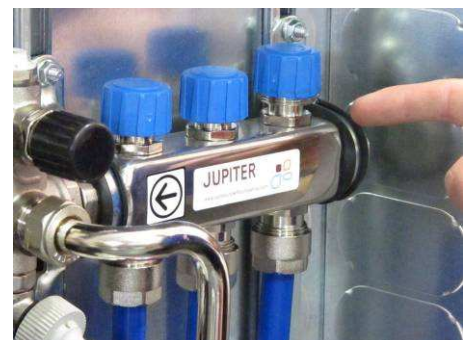
Screw down all blue caps on top valves except for circuit you wish to fill
