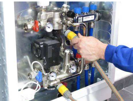
Fill via the lower valve and connect return hose to upper valve and allow to drain into an outside bucket.
