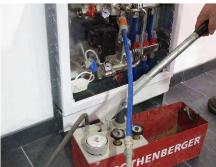
Once connected pump up to 8 bar. Once satisfied that there are no leaks, leave on test for a minimum of 1 hour. Once completed decrease pressure to 2 bar and then close return valve using cap. Release remaining pressure before removing test equipment from manifold. Remove hose and close cap. Re-open integral ball valves above and below pump.
