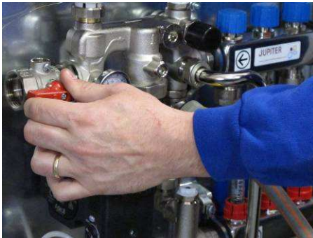
Close main flow and return isolating valves
