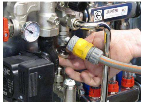
Once purged with air close fill & drain valves using cap. Close upper return valve first then lower fill valve. Only then turn off water supply and remove hoses.
