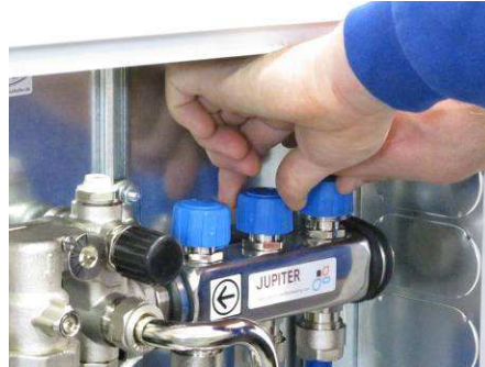
Once no more air bubbles emerge, simultaneously close the completed circuit and open the next one.
