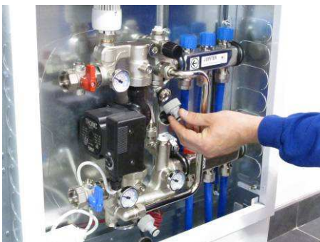
Attach hose lock adapters to upper and lower valves
