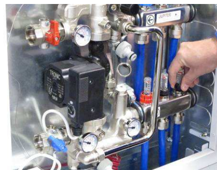
Take off red cap and fully open flow meters
