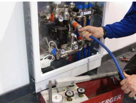
Re-open all blue caps on upper manifold prior to pressure testing. Connect pressure test equipment to upper return valve. Before connecting pressure test to the in-situ hose lock, pump some water out through the connecting pipe to avoid pumping more air into system. Before opening return valve with cap bring pressure up to approx. 5 bar.
