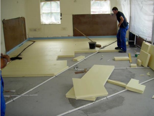
70mm ship lapped high density insulation being laid on levelled substrate.
