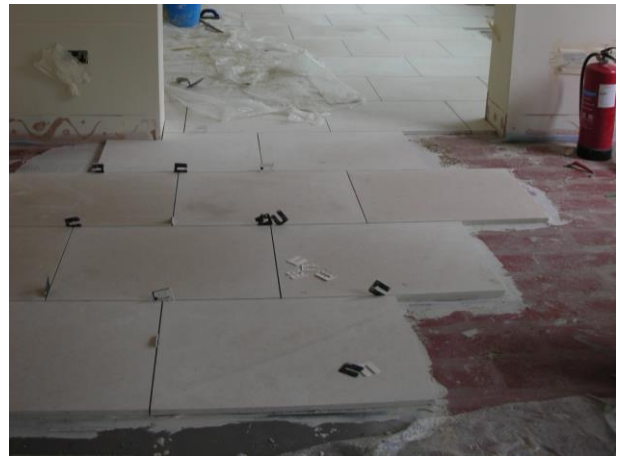
Large format 800 x 600 x 20mm limestone slabs being laid directly on the Screed Replacement Tiles
