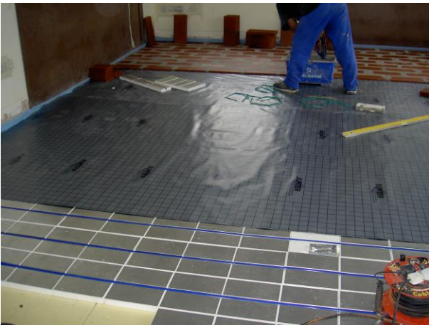
JUPITER Ideal panels laid directly on the high density insulation.
