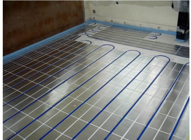
Once in position, pipes are clipped into the tracked panels.
