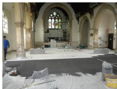
Levelling of slate using levelling bars
