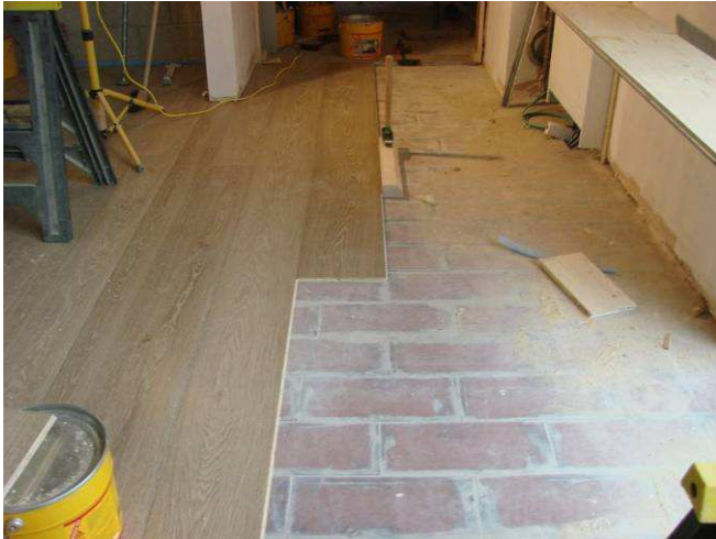
Screed Replacement Tiles installed as a floating floor over the JUPITER IDEAL EPS system.
