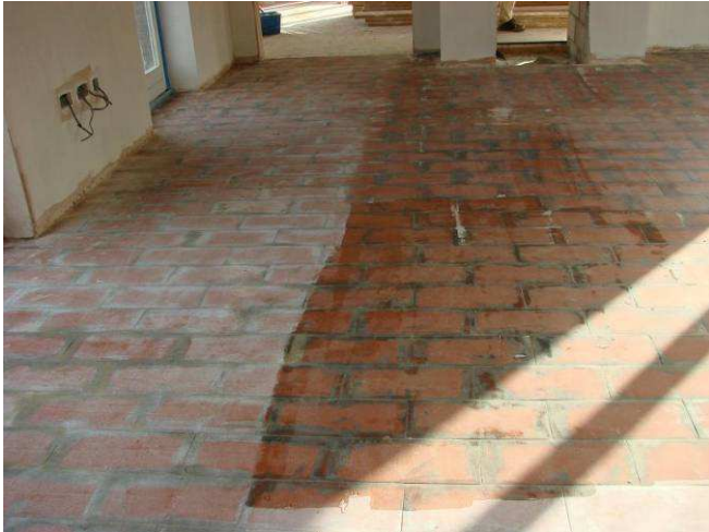
Screed Replacement Tiles installed as a floating floor over the JUPITER IDEAL EPS system.
