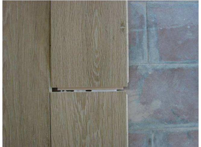
T&G ends of timber are fixed using wood adhesive.
