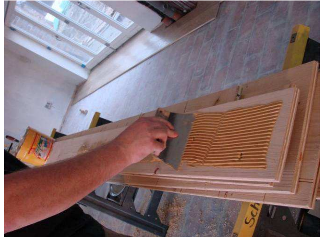
Schotten & Hansen engineered timber floors being prepared for gluing to Screed Replacement Tiles with Sikabond T-54.
