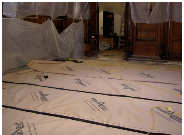
Height available for the heating system and finished floor was approx. 85mm.
