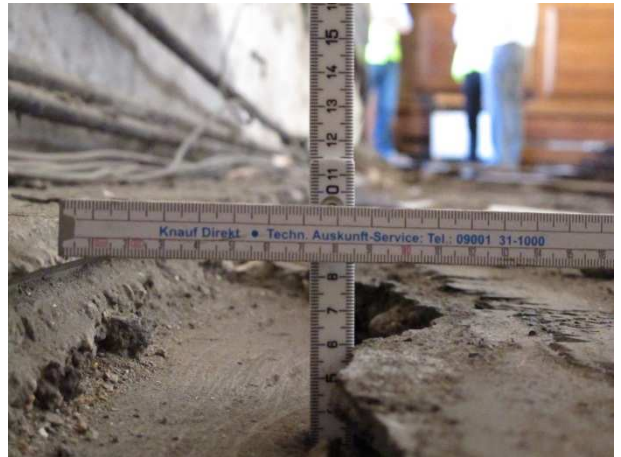
Height available for the heating system and finished floor was approx. 85mm.
