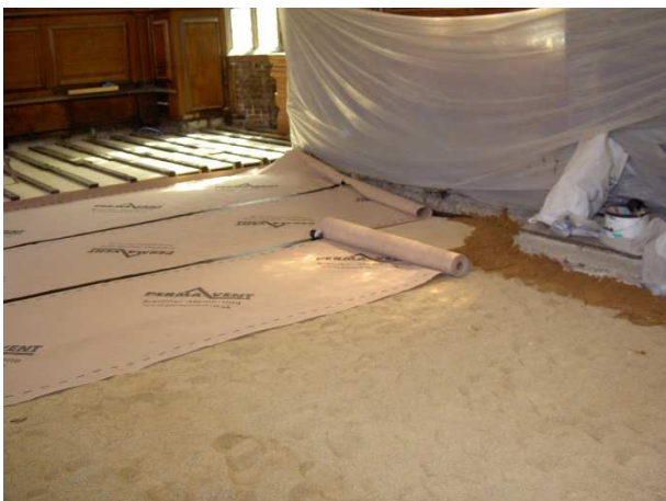
A layer of sharp sand was installed
