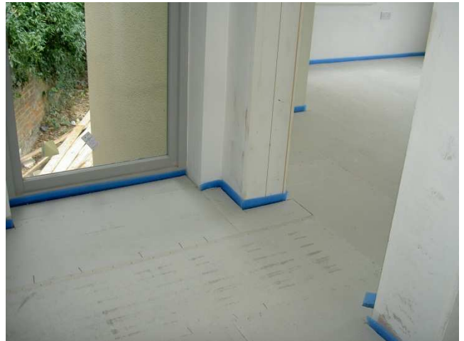
20mm Fermacell 2E11 installed as load bearing surface in carpeted bedrooms.
