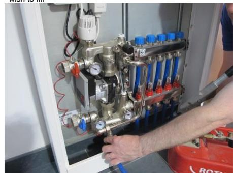
Re-open all blue caps on upper manifold prior to pressure testing. Connect pressure test equipment to upper return valve. Before connecting pressure test to the in-situ hose lock, pump some water out through the connecting pipe to avoid pumping more air into system. Before opening return valve with cap bring pressure up to approx. 4 bar.
