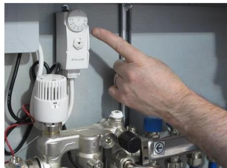
240v temperature limit thermostat is factory set to 60°C. Do not make unqualified adjustment.
