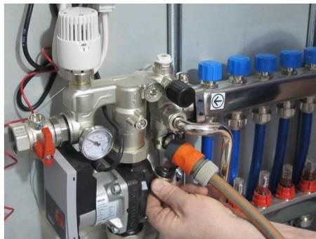
Once purged with air close fill & drain valves using cap. Close upper return valve first then lower fill valve. Only then turn off water supply and remove hoses.
