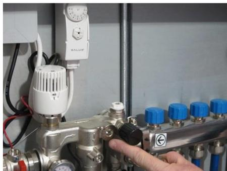
Do not adjust the primary water temperature regulator. The factory setting is 3. The unit is delivered with the black bypass knob closed. Once system is filled open by 1/16 of a turn anti clockwise. This allows water through the blending valve in the event that all circuits are closed.
