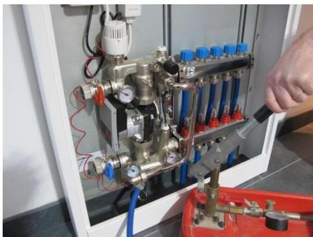
Once connected pump up to 6 bar. Once satisfied that there are no leaks, leave on test for a minimum of 1 hour. Once completed decrease pressure to 2 bar and then close return valve using cap. Release remaining pressure before removing test equipment from manifold. Remove hose and close cap. Re-open integral ball valves above and below pump
