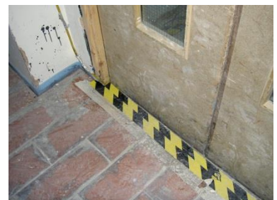
Do not apply loads at edge of system. Warning tape should be used
