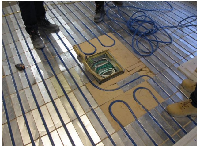
IDEAL ECO installed to provide acoustic insulation
