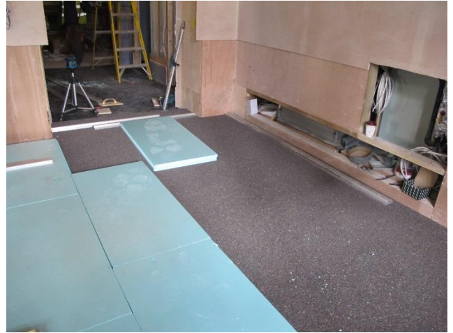
Existing slabs levelled with dry levelling slate
