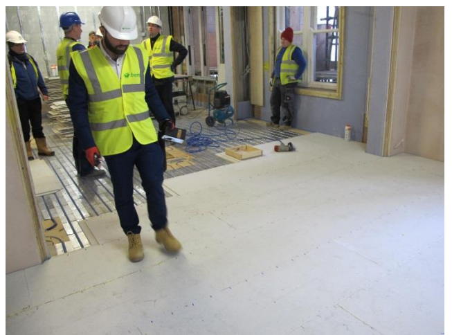
Fermacell installed in timber / carpeted areas
