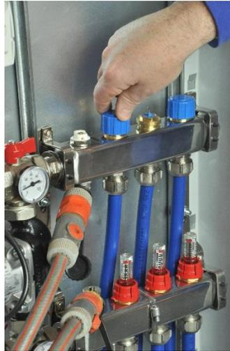
Once no more air bubbles emerge, open next circuit and use blue cap to close previous circuit.
