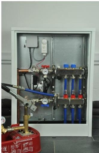
Attach pressure test to lower fill valve. Open lower fill valve with attached key and test pressure to 6 bar. Once satisfied there are no leaks leave on test for a minimum of 1 hour.
