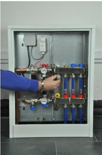
Attach Hozeolock fittings to fill and drain valves
