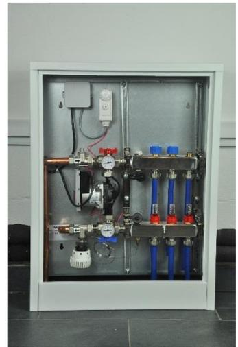
Remove blue cap from lower 2 port valve and replace the thermostatic valve. Recommended setting is set point 4.5 (see table below)
