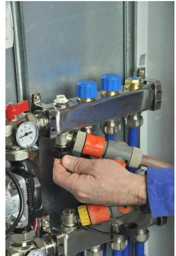
Once all circuits are purged, close fill and drain valves using cap. Close upper return valve first then lower fill valve. Only then turn off water supply.
