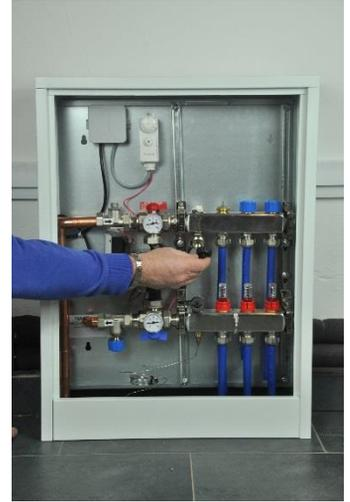
Remove filler cap to use as valve key
