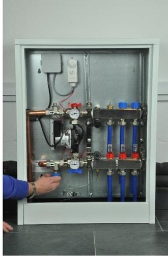
Replace with blue cap from top valve and tighten
