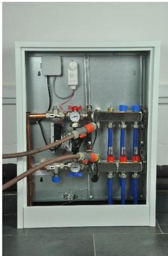
Attach fill (lower) and return (upper) hoses and turn on water supply. Allow to drain in to bucket.
