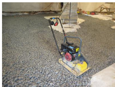
Foam glass can be gently compacted with a lightweight vibrating shovel compactor
