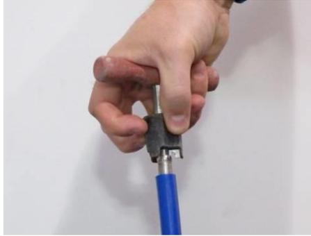
Always deburr the end of pipe with bevelling tool before attaching to manifold
