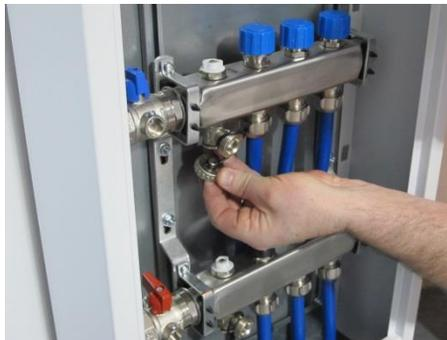
Open fill and drain valve using key on the back of cap
