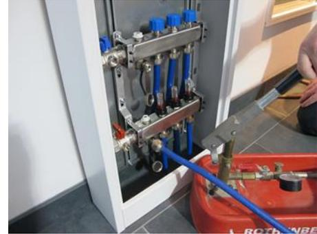
Once connected pump up to 6 bar. Once satisfied that there are no leaks, leave on test for a minimum of 1 hour.
