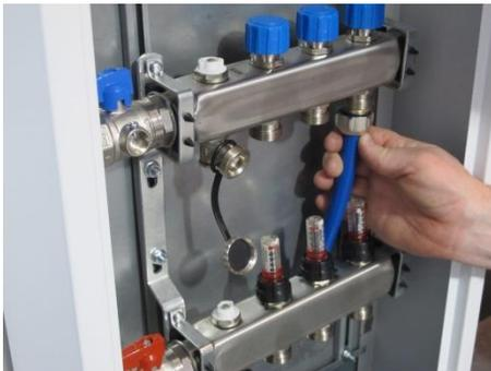
Push Eurokone insert and pipe into manifold and tighten up with spanner
