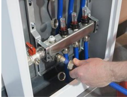
Connect pressure test equipment to upper return valve. Before connecting pressure test pump some water out through the connecting pipe to avoid pumping unnecessary air into system. Before opening return valve with cap bring pressure up to approx. 4 bar
