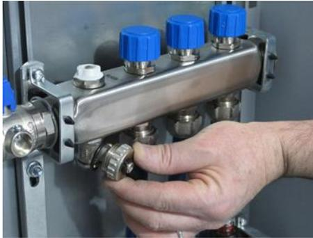
Once completed decrease pressure to 2 bar and then close return valve using cap. Release remaining pressure before removing test equipment from manifold. Remove testing equipment and close cap.
