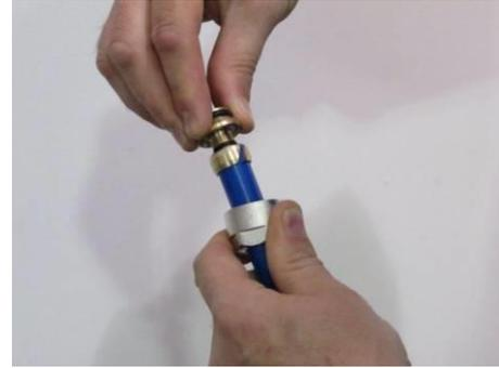
Place nut and brass split ring over pipe before inserting Eurokone fitting
