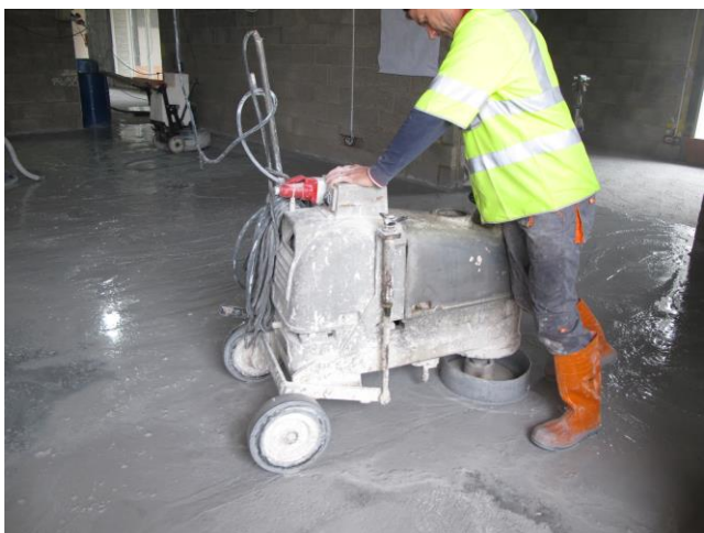
Grinding process of terrazzo floor
