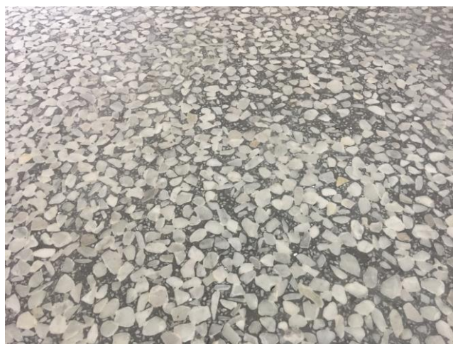
Finished ground terrazzo
