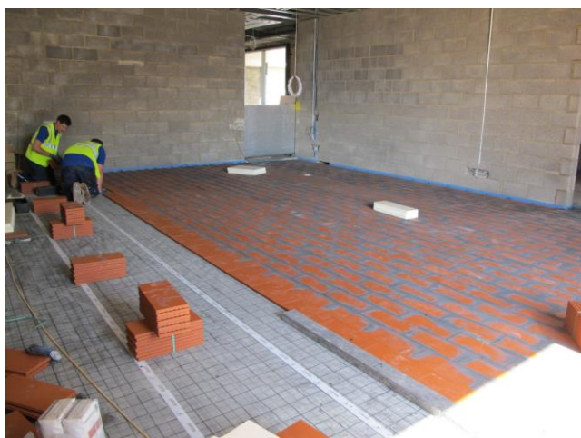
Screed Replacement Tile installed over UFH
